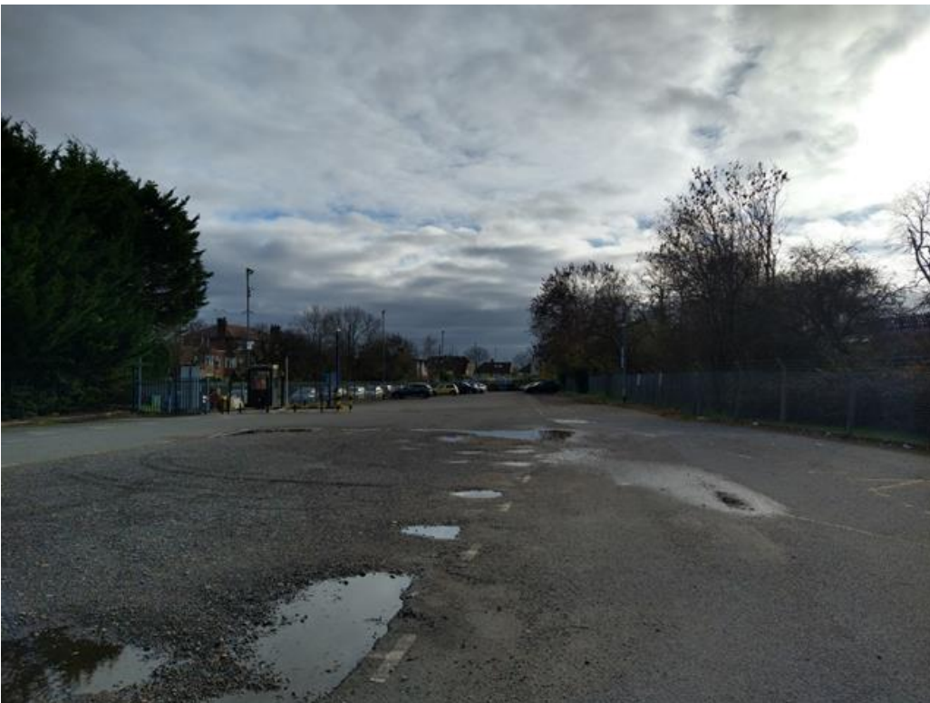
View of the station car park facing south
