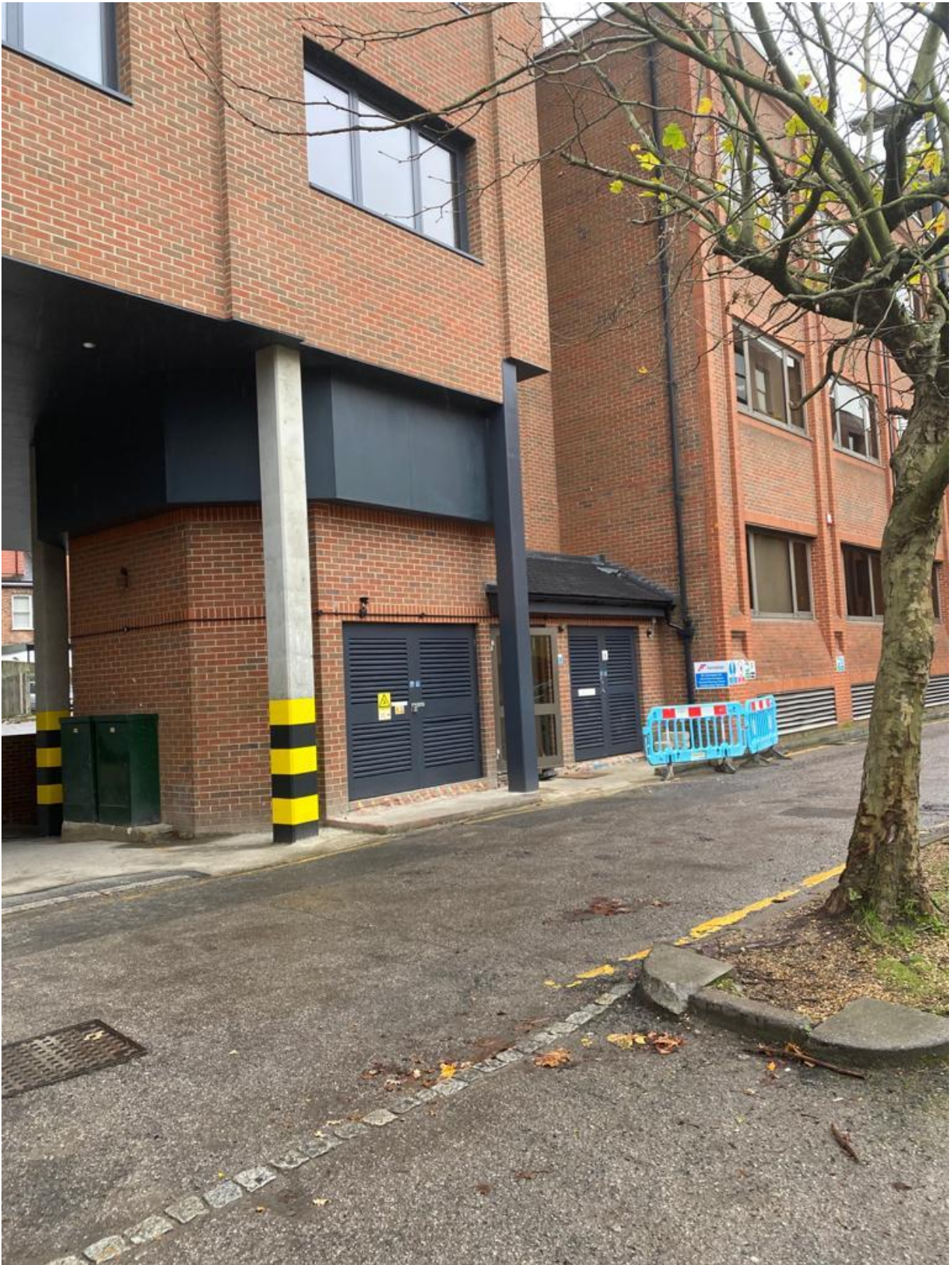
Proposed new location for some bins / existing substation location
