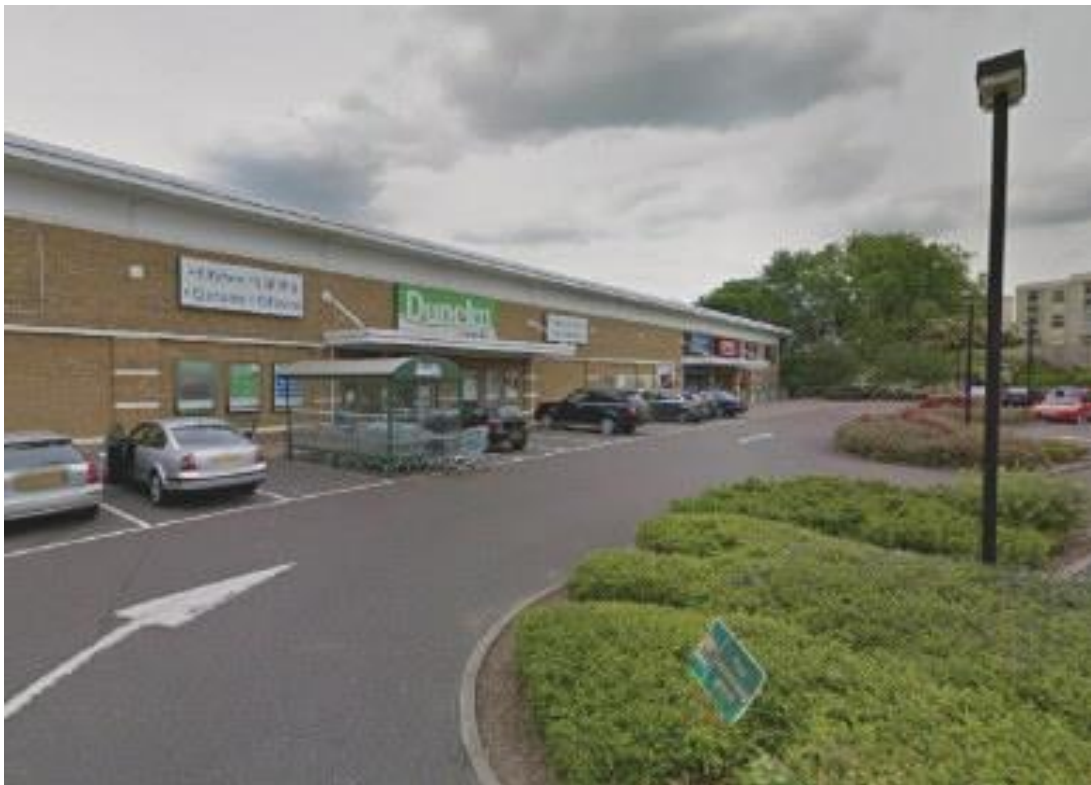
View of site from car park of retail park
