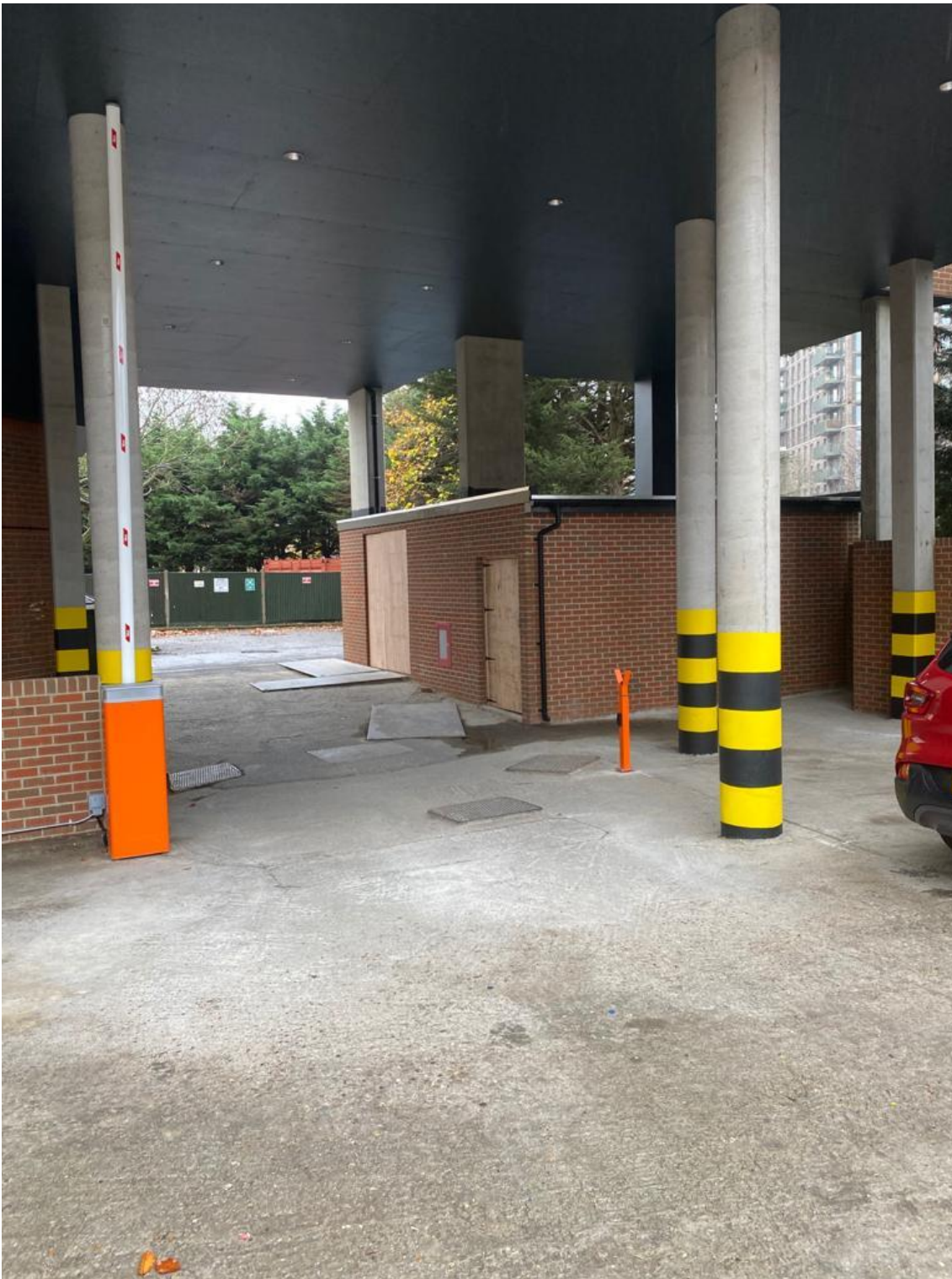
Outbuilding, as currently on site
