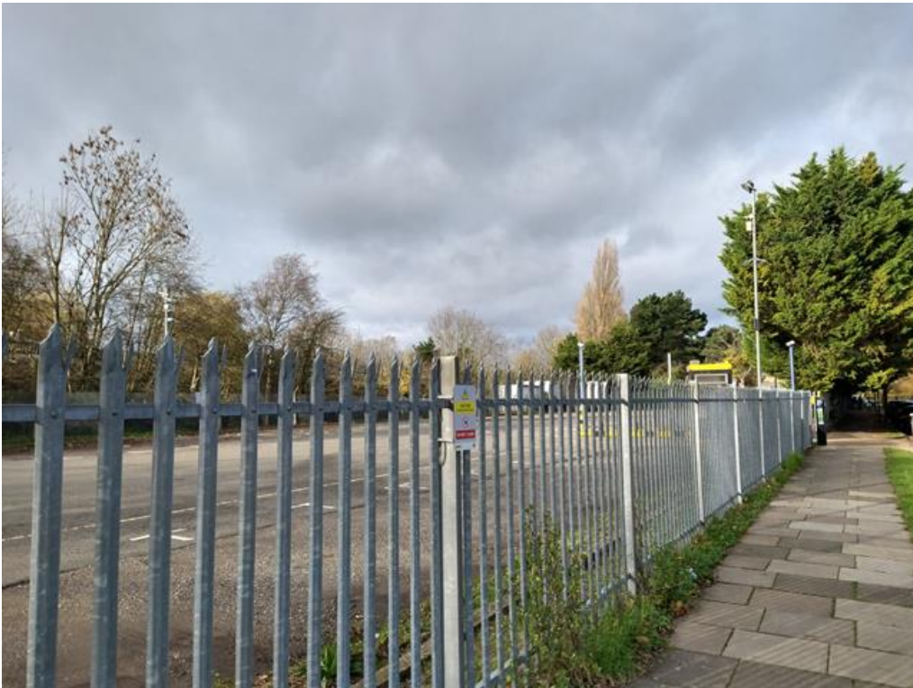
View of the station car park from the pedestrian footway
